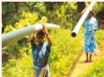
Transportation of pipes by manual head load to DBI site, PRAGATI.
