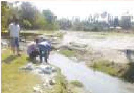
Auto Level survey work at SeSTA DBI site, Assam
